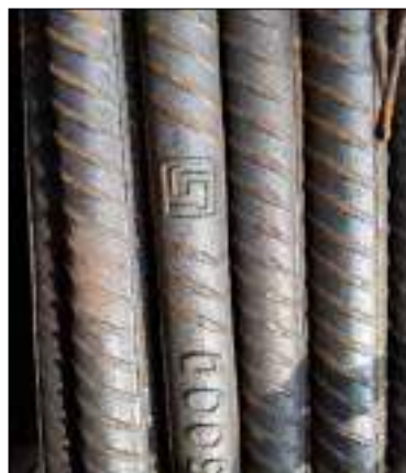
Fig. 1. Fresh ribbed bars showing start of corrosion at damaged ribs
