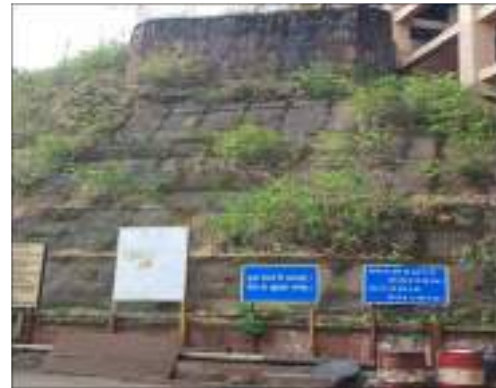
Figure 2. Front view of Blanket wall benches
