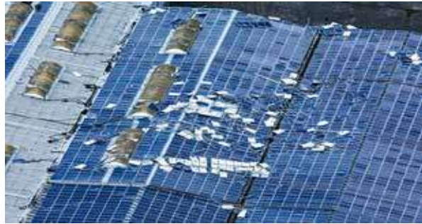
Fig 1. Damaged solar panels due to high wind over the hipped roof [3]
