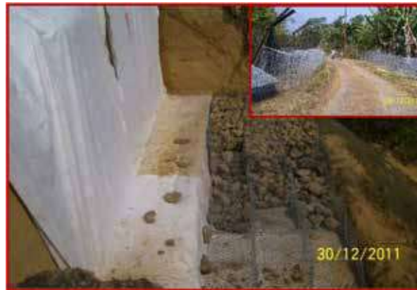
Plate 3 : A rock fill gabion wall with geotextile backing under construction. Inset : Gabion boxes being prepared for placement.
