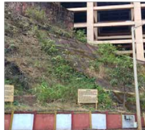
Figure 4. Side view of Blanket wall
