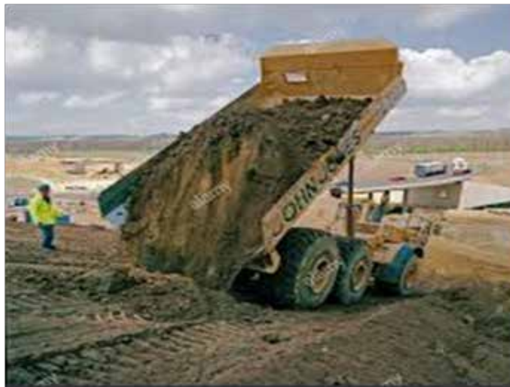
Fig. 2. Restoration of topsoil
