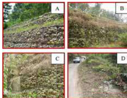
Plate 5:[A] May 2012 – Some green cover is seen over the gabion walls [B] March 2013 – Green cover has increased [C] March 2013 – Soil fill gabion panels are holding fine [D] February 2015 – No subsidence is seen at wall location. Vegetation growth is abundant
