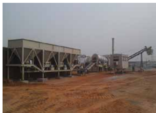
Fig. 1(b) Real image of drum mix plant
