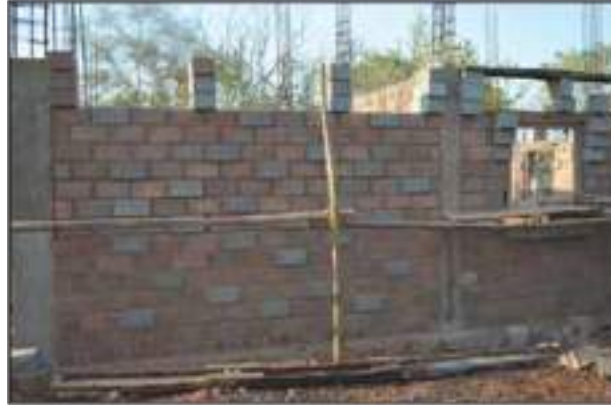
Fig. 11. Construction of two story house using LC 3 [14]
