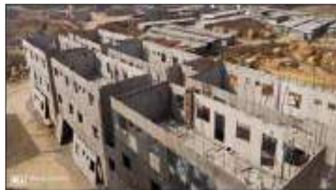
Fig. 4: Construction of 1512 DUs in S+S+9 Pattern at Dundigal using Precast Technology
