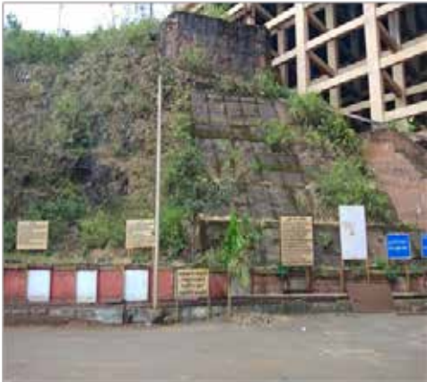
Figure 1. Front view of Blanket wall
