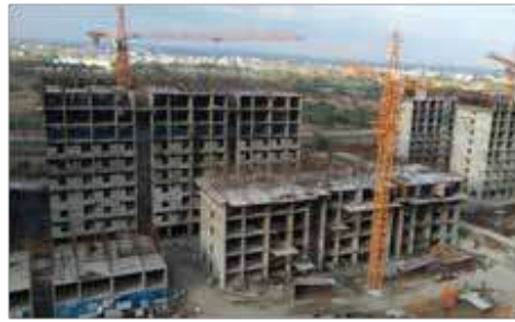
Fig. 3: Construction of 6240 DUs in S+10 Pattern at Rampally with Shear wall Technology - Tunnel Form Work
