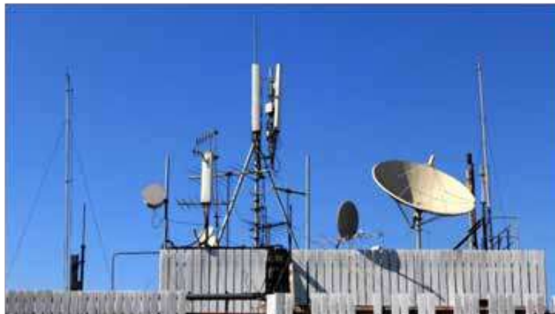
Fig. 2. Multiple antennas closely mounted at control station
