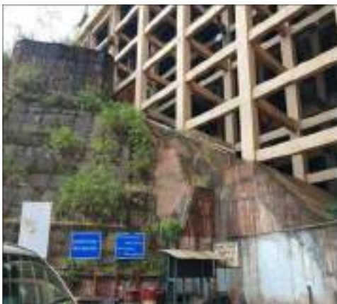
Figure 3. view of Blanket wall at primary crusher entry
