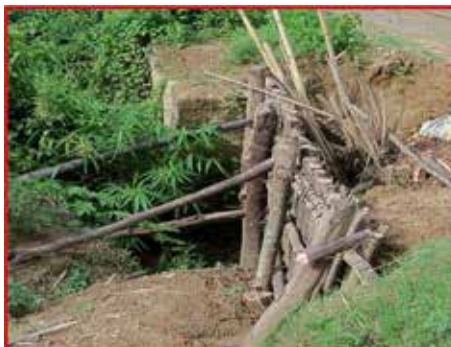
Plate 2 : Bamboo / wooden piles with inclined stays and bamboo mat behind them to retain the earth. A brick masonry retaining wall is also seen in the background.
