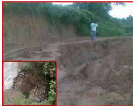
Plate 1 : Extensive damage to IBB road in Tripura – The soil subgrade has been totally eroded and rain water has made deep channels on the road side. Inset : Damage to random rubble masonry retaining wall.
