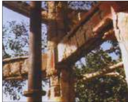
Fig. 2. Distress in staging of overhead water reservoir due to corrosion in rebars
