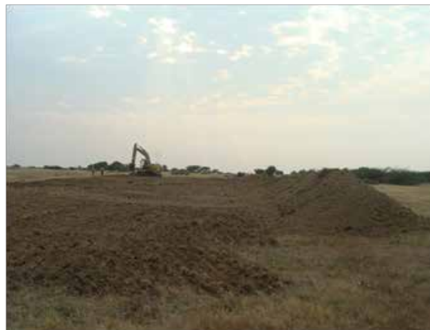
Fig. 1. Stripping of topsoil
