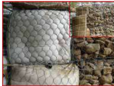
Plate 4 : Soil filled Gabion wall provided with HDPE drainage pipe as an additional drainage measure. Inset : Use of bamboo mat for UV protection
