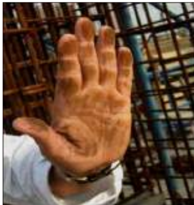
Fig. 4. Ribbed bars coated with products of corrosion even before concreting, leading to a total loss of bond with concrete
