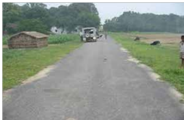
Fig. 1. PMGSY Road – Poor Maintenance
